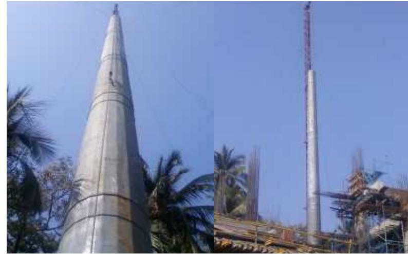
Erection of 72 mtr Highmast with the help of Derrick arrangement due to acute space constraints at Wankhede Cricket Stadium, Mumbai for the World Cup, 2011.
