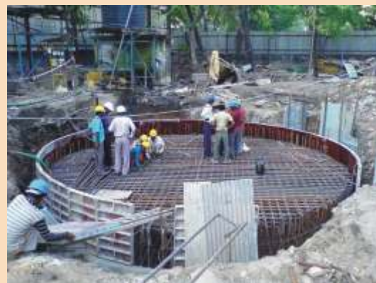
Foundation of the Mast
