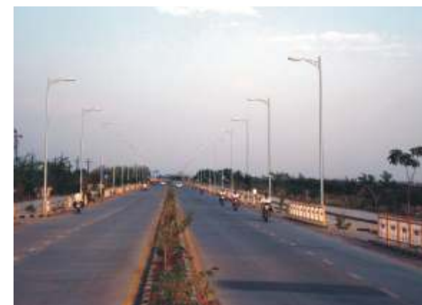
Street Lighting at Municipal Corporation, Nanded.
