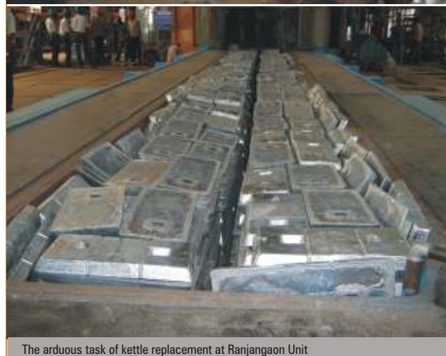
The arduous task of kettle replacement at Ranjangaon Unit
